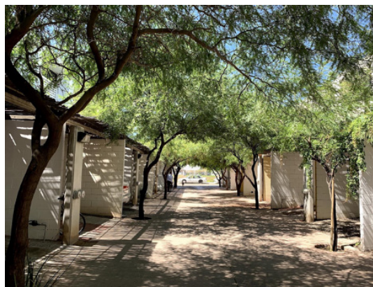
Figure 3. Exterior of houses in the Bosco Development
